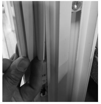
**STEP ONE:** To access wafer head jamb adjuster, lift lower exterior edge of balance cover side corners. Once started, it can be unlocked by slding finger up jamb between cover and jamb.
