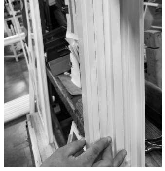
**STEP FOUR:** To replace balance covers position covers over jambs with interior edge of covers in balance cavity. Relocate by folding lower exterior corners into place and sliding finger up joint.
